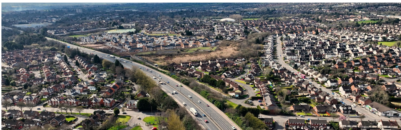
M1 Motorway Southbound Dublin Road Westlink Belfast City
