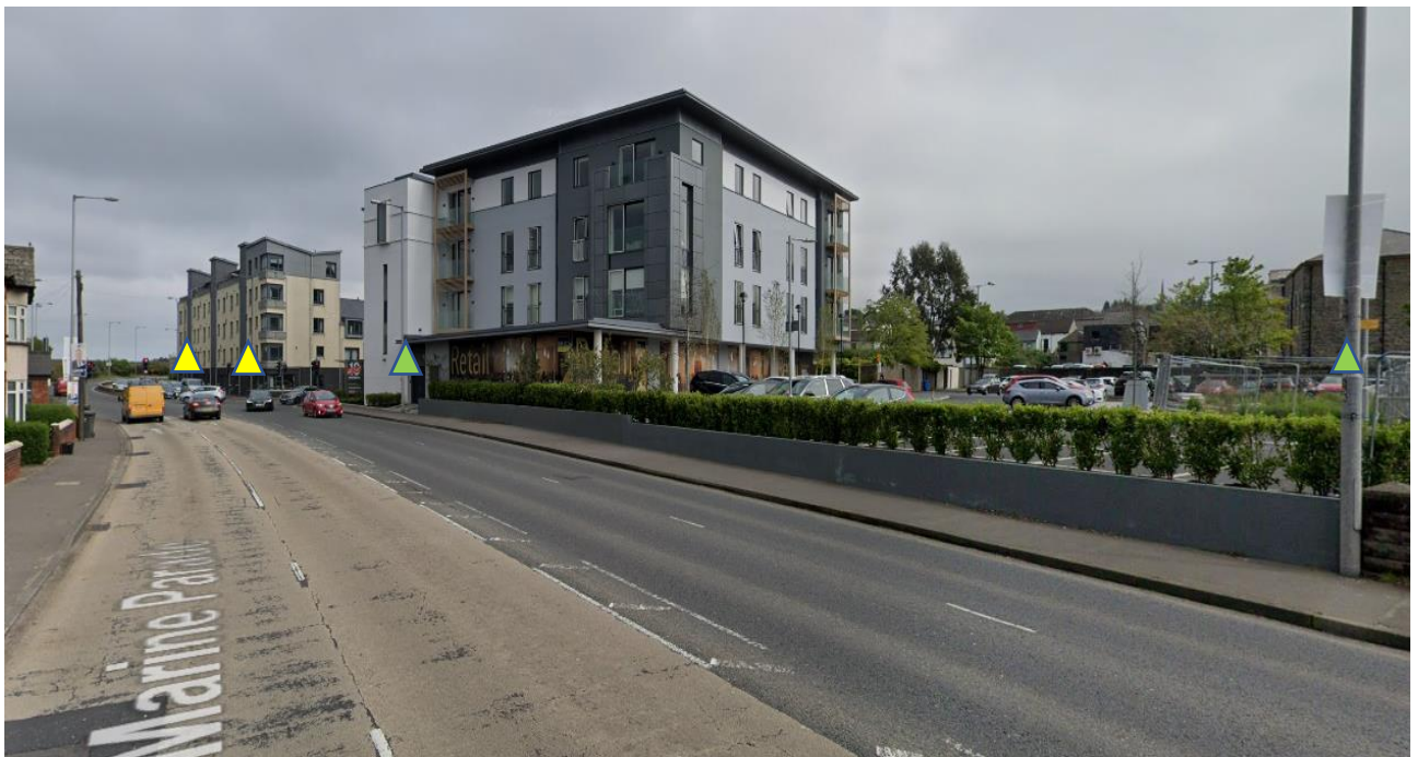
Figure 2.11 Holywood junction A2
